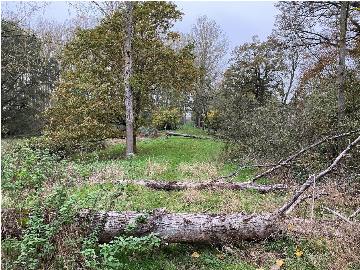
Plate 1 General view along crest of dam, from east end looking northwest, showing trees on dam slopes and in reservoir, which is on left-hand side.
